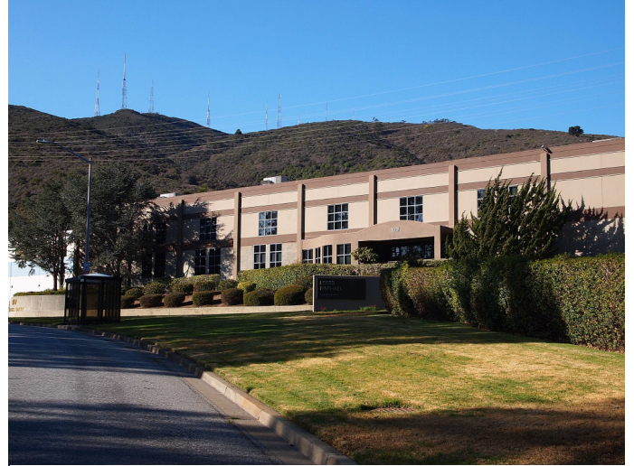
The Louis Raphael facility is located at the Intersection of West Hill Boulevard and West Hill Place and workers have Bay Views over Crocker Park
